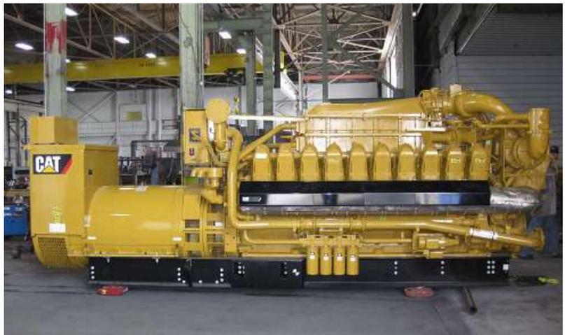
*The generator set was sized to meet the majority of the buildings electrical load and to supplement the original heating and air conditioning systems.*
